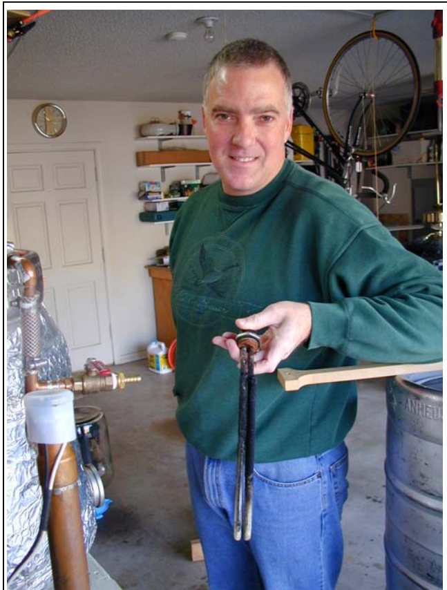
Don't find yourself on the wrong side of this water heater element.
